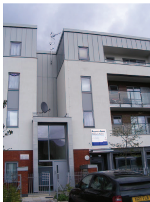
Picture 4.9 Making an Entrance! But note the poorly sited satellite dish and television aerials
